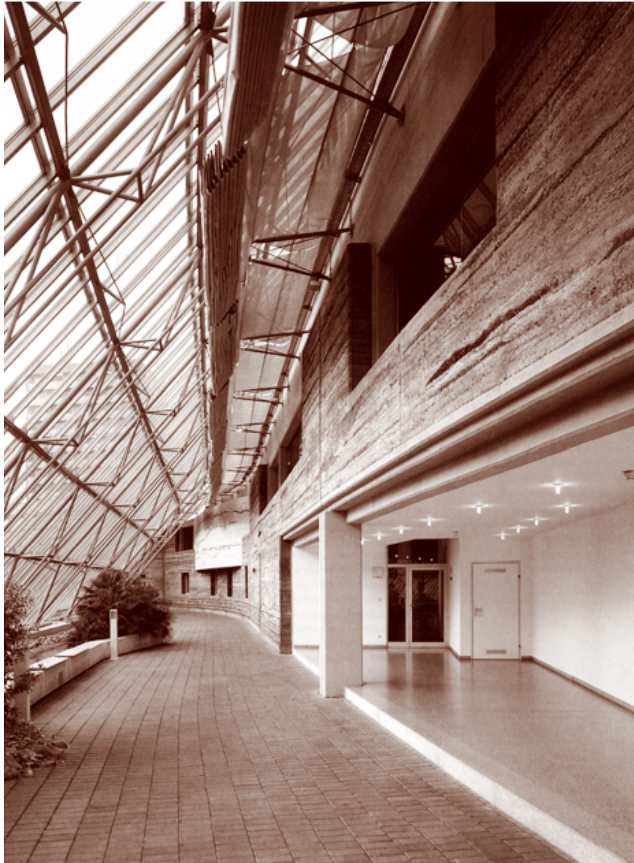
Martin Rauch's rammed earth wall at Feldenkirch Hospital, Austria
