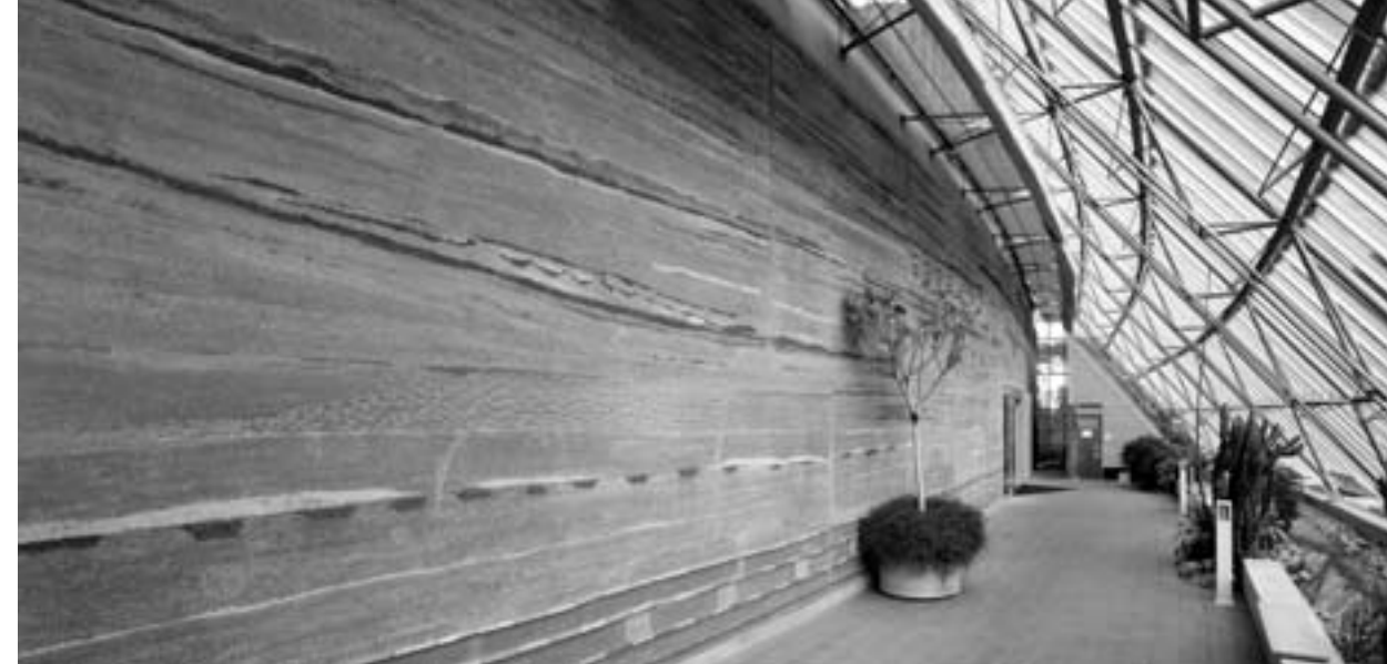
Closer view of the rammed earth wall at Feldenkirch Hospital, Austria.
